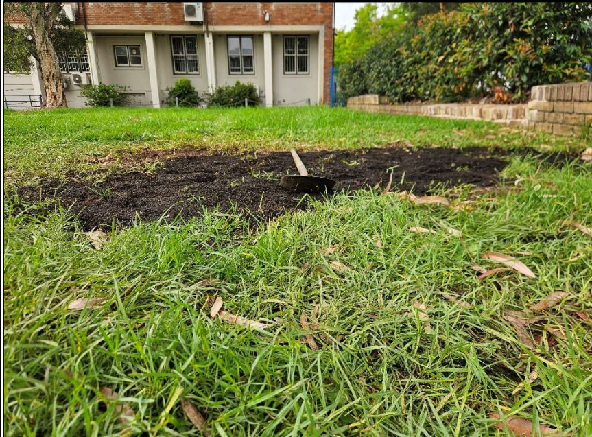
PHOTO 27: REINSTATEMENT OF TP103 SURFACE FINISH (TOPSOIL) IN THE WEST OF SITE
