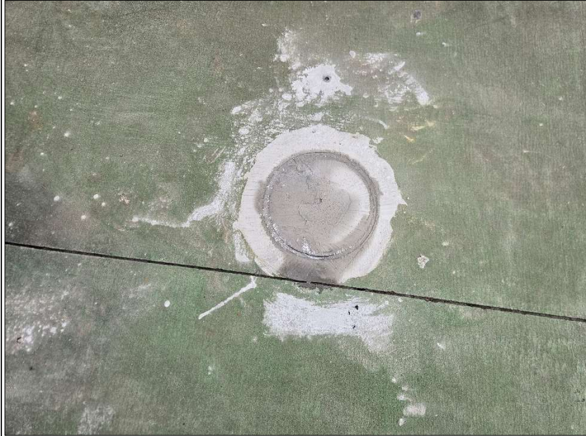
PHOTO 28: REINSTATEMENT OF BH103 SURFACE FINISH (SYNTHETIC TURF) IN THE NORTH OF SITE
